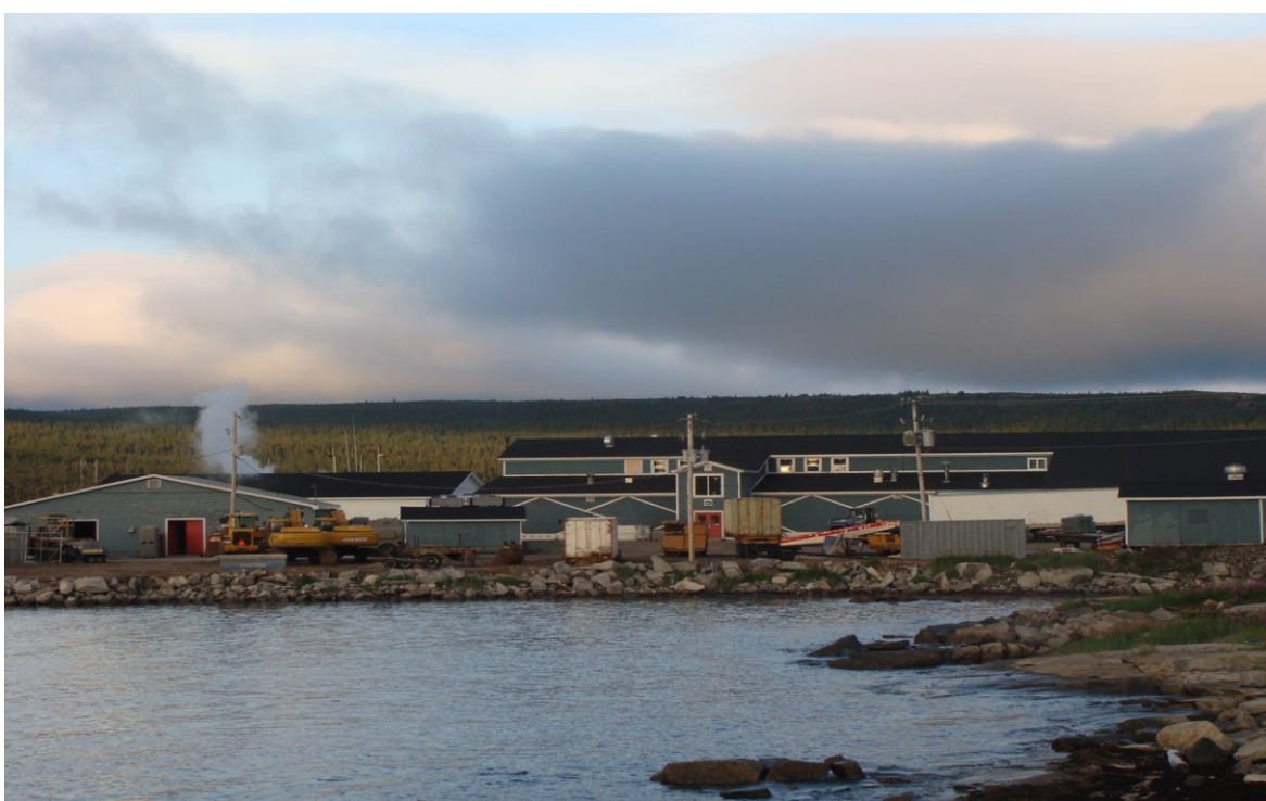
Fig. 18: Fish Processing Plant in Makkovik
