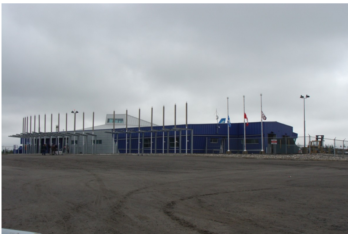
Fig. 13: New Kuujjuaq Airport 2008
