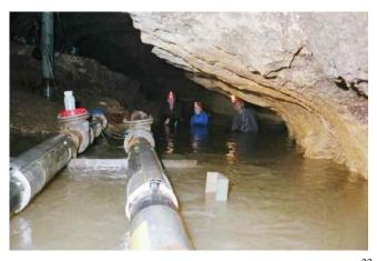
Figure 7.20. Groundwater pumping in Bribin cave<sup>22</sup>
