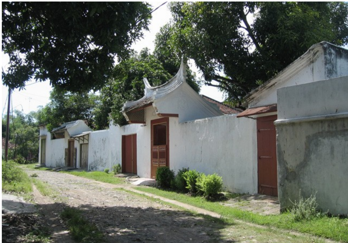
Picture 6: Chinese style house from outside with characteristic walls in Lasem (15.04.2010).
