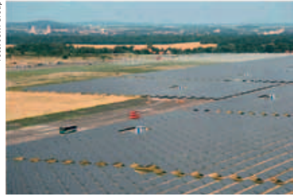
Image 6: In Waldpolenz-Solarpark near Leipzig, the world's largest thin-film photovoltaic facility is being constructed and consists of cadmium-telluride thin film cells.
