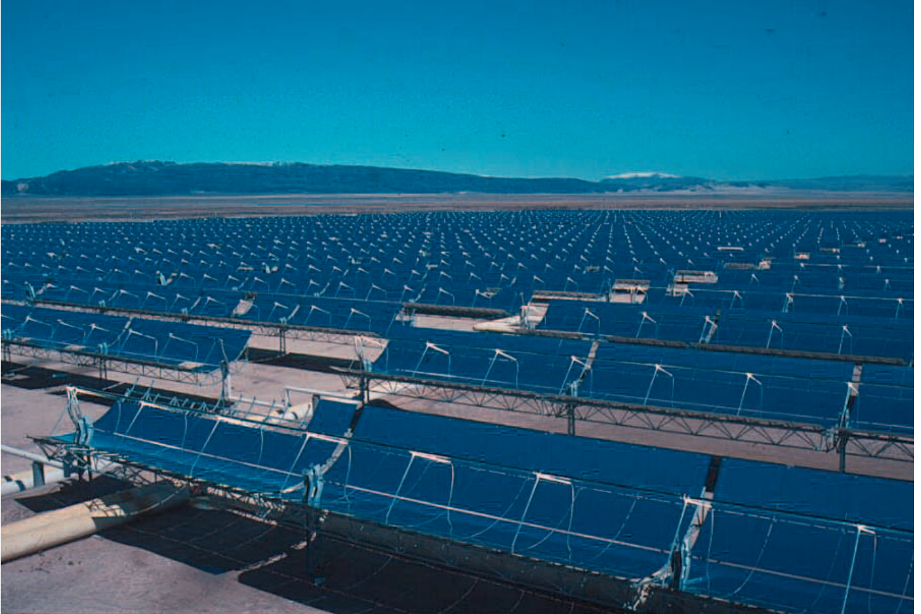
Image 1: Large solar power stations in the desert regions of the earth (seen here in California/USA) are capable of securing humanity's long-term energy requirements. A solar power parabolic trough system uses cylindrical mirrors to concentrate sunlight onto absorber tubes. The heat created is transferred to a steam plant and generates electricity.
