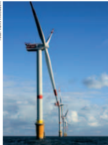
Image 4: As the winds are stronger on the open seas than on the land, it makes good sense to set up offshore wind farms despite the higher investments and maintenance costs. Each of the rotors, located off of the Belgian coast has a diameter of 126 m and a capacity of 5 MW.
