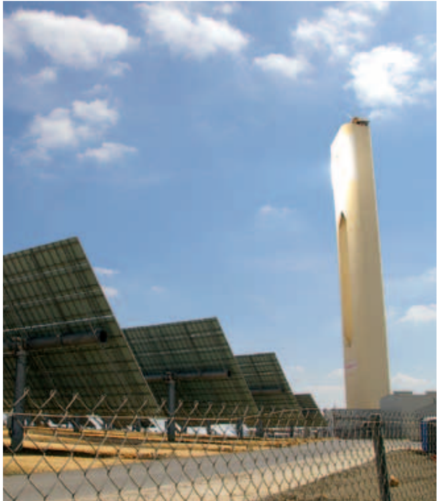
Image 2: Solar tower power station PS10 near Sanlúcar la Mayor, west of Seville. 120 mirrors focus sunlight onto a 115 m high tower. In this way 6,000 homes are supplied with electricity.
