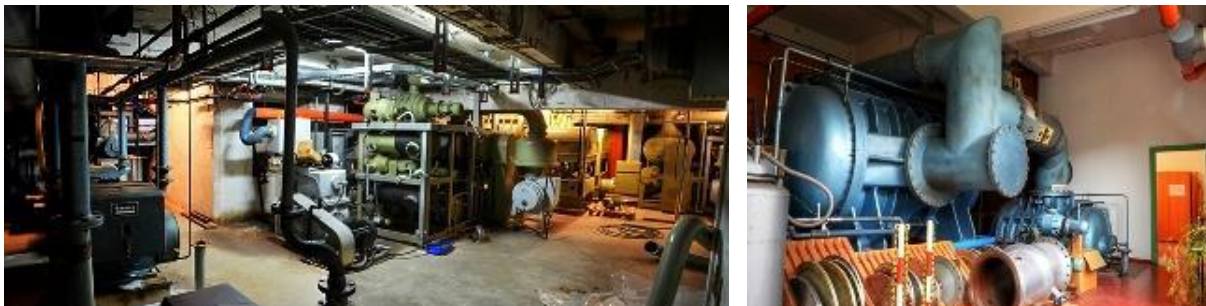
Fig. 16: Picture of vacuum pump facility in cellar with 21 pumps (left), picture of biggest vacuum pump in front compared to 2 m high door (right)
