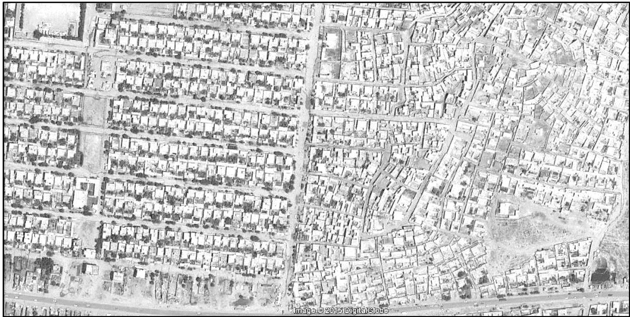
Figure 27: Difference in layout of roads and right-of-way between formal and informal settlements
