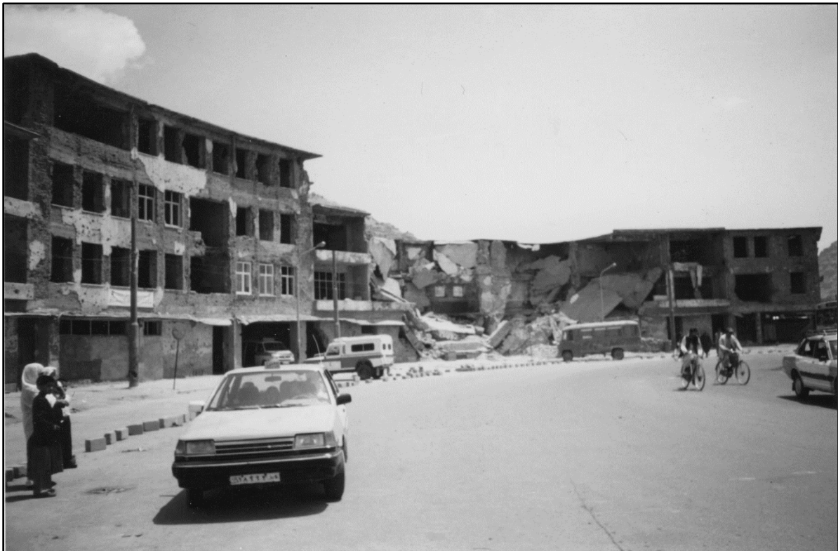
Figure 12: The ruined building of Kabul Traffic Department in 2003. The damaged buildings have been reconstructed, while the damaged institutions are still in need of rehabilitation.
