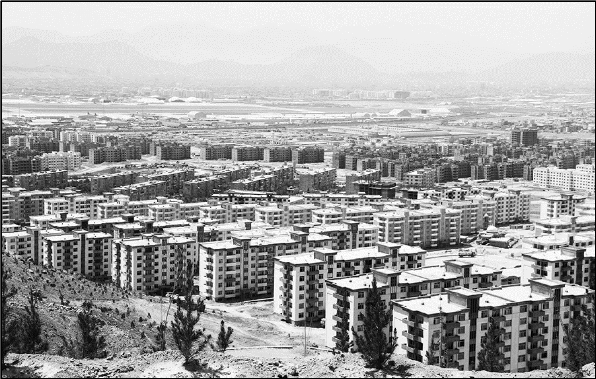
Figure 23: Khwaja-Rawash, the largest public-private housing project in the country Photo Source: KHAMA PRESS (2016)
