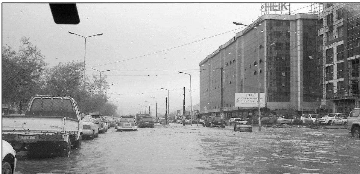
Figure 24: Water blockage due to deficiency of surface water drainage system in Kabul Photo: SAYED 2010
