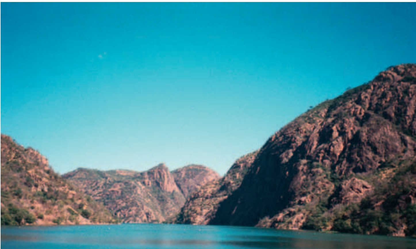
Cabora Bassa Dam at the Zambezi River in Mozambique, one of the most controversial mega-energy projects in Africa.
