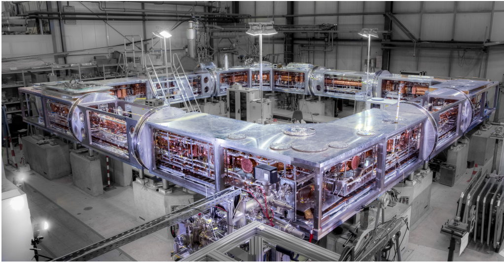
Figure 3.5.: Photography of CSR during preparation of the room-temperature commissioning phase in spring 2014. At this point, the isolation vacuum chamber was still open, showing the copper-wrapped beam-guiding vacuum chamber. During commissioning, the outer chamber was closed in order to provide safe high-voltage operation. Since the thermal shields were not yet completely installed at this time, the storage ring could not yet operate in cryogenic mode.
