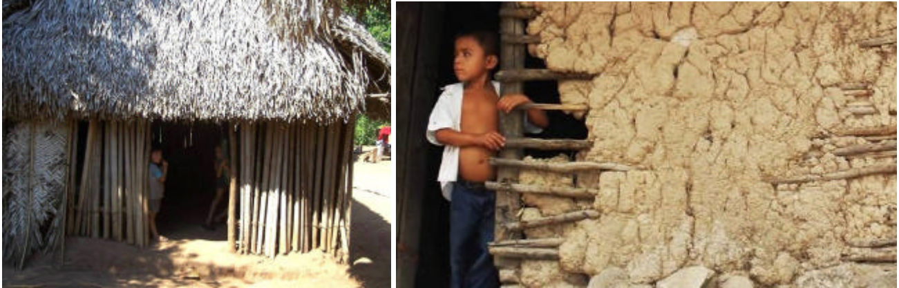
Figure 1.6-2 Palm house in El Beni, Bolivia (left) and "adobe" house in Guatemala. These kinds of dwellings are characteristic of low-income settlements. Triatomine bugs live in the palm roofs and in crevices of adobe houses, getting out, mainly at night, to feed blood from sleeping people. (Image left: courtesy of Beck E; right: Médecines Sans Frontières, MSF).
