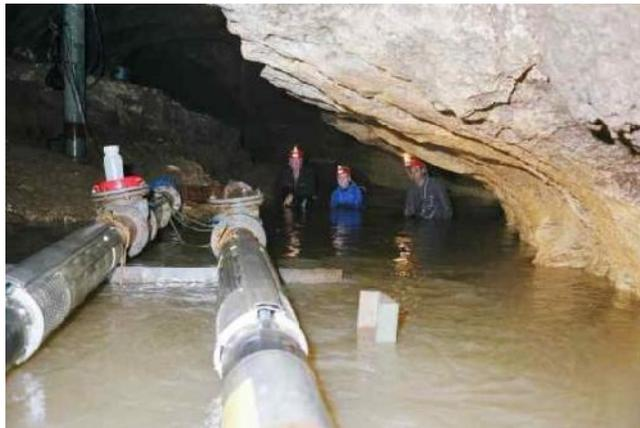
Figure 7.20. Groundwater pumping in Bribin cave<sup>22</sup>
