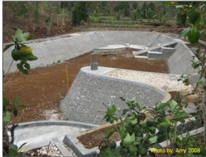
Figure 4.12. Cemented wall Karst Pond in Tepus sub-district, which in turn shortens the rain water holding period
